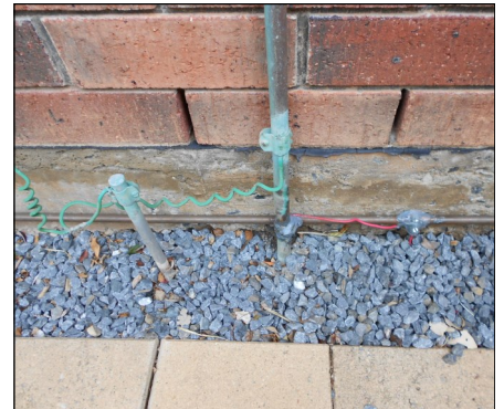
← Several radials bonded to the workshop shed as above. Note a pair of radials run in the paving slab channel and smothered with silicone: these head out to the opposite side of the yard boundary fenceline for about 165ft.
