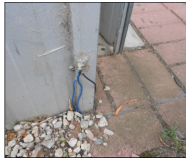
← Several radials bonded to the workshop shed as above. Note a pair of radials run in the paving slab channel and smothered with silicone: these head out to the opposite side of the yard boundary fenceline for about 165ft.
